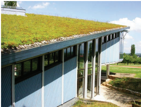
Figure 16: An extensive green roof of meadow grasses in Stuttgart, Germany (Photo: N. Williams).
