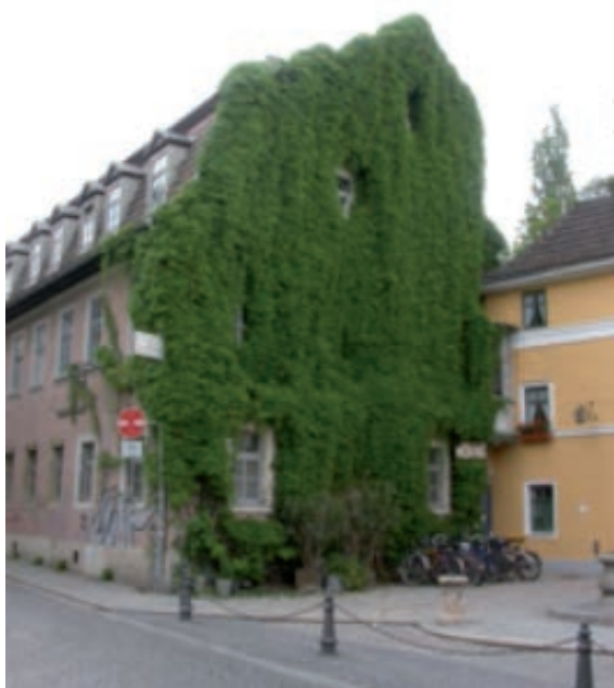
Figure 17: A green facade of Virginia Creeper, in Weimar, Germany (Photo: N. Williams).
